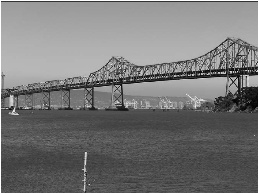
Figure 1. The old Bay Bridge is being replaced with new seismic engineering.
